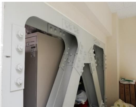
Braces inside the building
