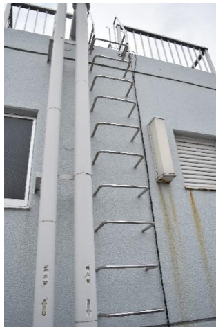
Aluminum fence and stairs
