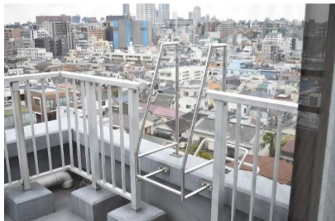
Stainless steel stairs leading up to the penthouse
