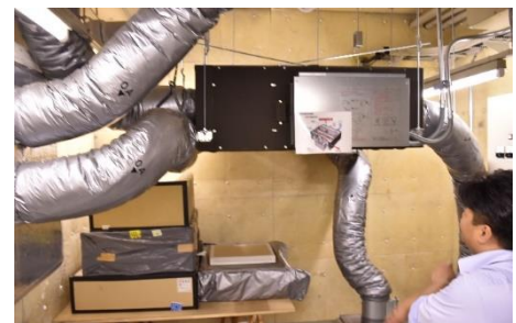
Desiccant air conditioning that pursues the comfort of tenants
