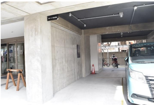
Earthquake-resistant walls and a column covered with aramid fibers on the 1 st floor (left)
