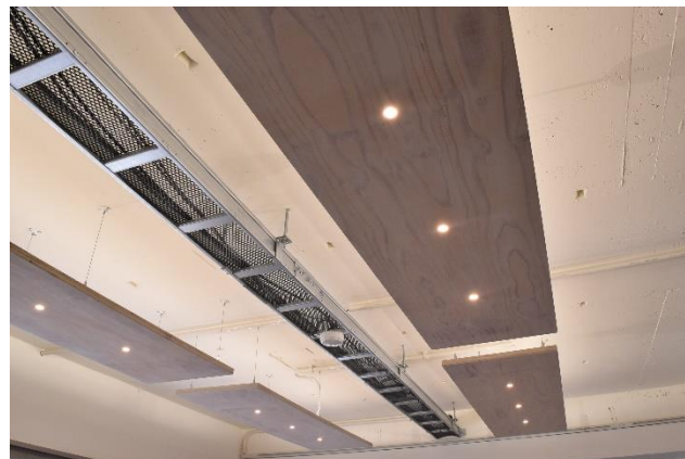
The suspended ceilings were removed, and the indirect lightings were attached directly to the ceiling.
